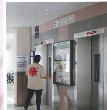
Upgrading of Lift Lobby at Zone G (Blks 748 to 760, 762 to 763 Woodlands Ave 4, Circle)
