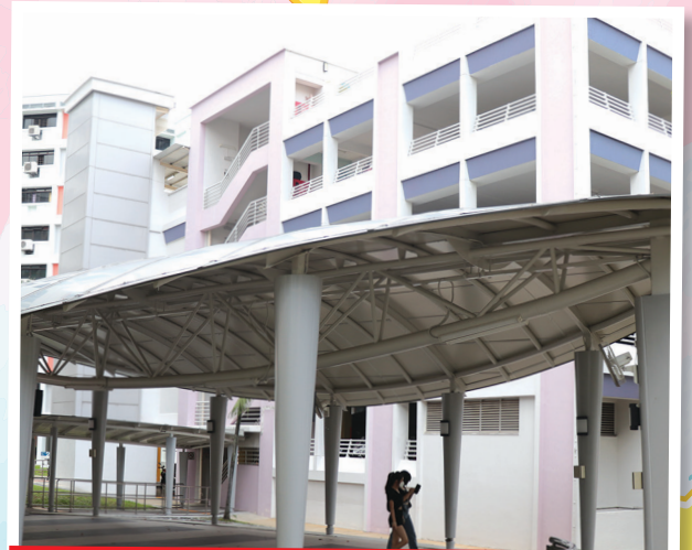
Upgrading of Existing Covered Walkway and Link Building Between Blk 605/605A to 605B Woodlands Drive 42 (Link Building)
