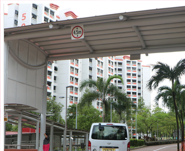
Construction of High/Low Linkway at Blk 501A Wellington Circle
