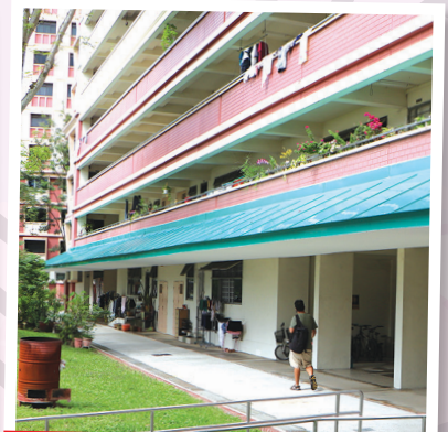
Construction of Awning at Blk 302 Canberra Road
